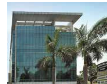
SHALIMAR LOGIX RANA PRATAP MARG LUCKNOW
