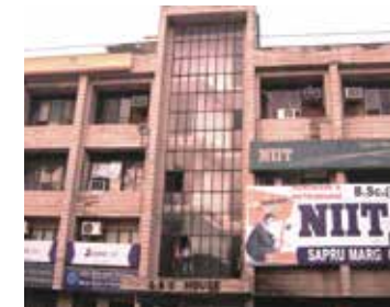
SAS HOUSE SAPRU MARG LUCKNOW
