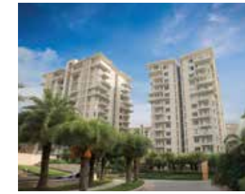
SHALIMAR GALLANT MAHANAGAR LUCKNOW UPRERAPRJ3168
