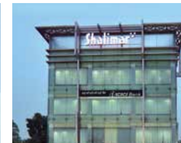
SHALIMAR STAR, HAZRATGANJ, LUCKNOW
