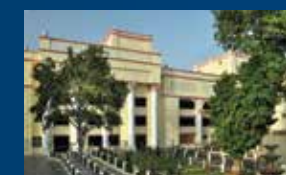
Multilevel Parking, Hazratganj, Lucknow
