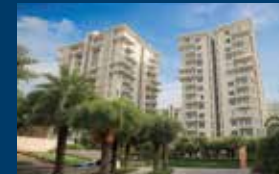
Shalimar Gallant, Mahanagar, Lucknow UPRERAPRJ3168
