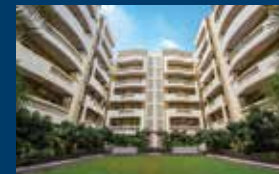
Shalimar Dwelling, AP Sen Road, Lucknow
